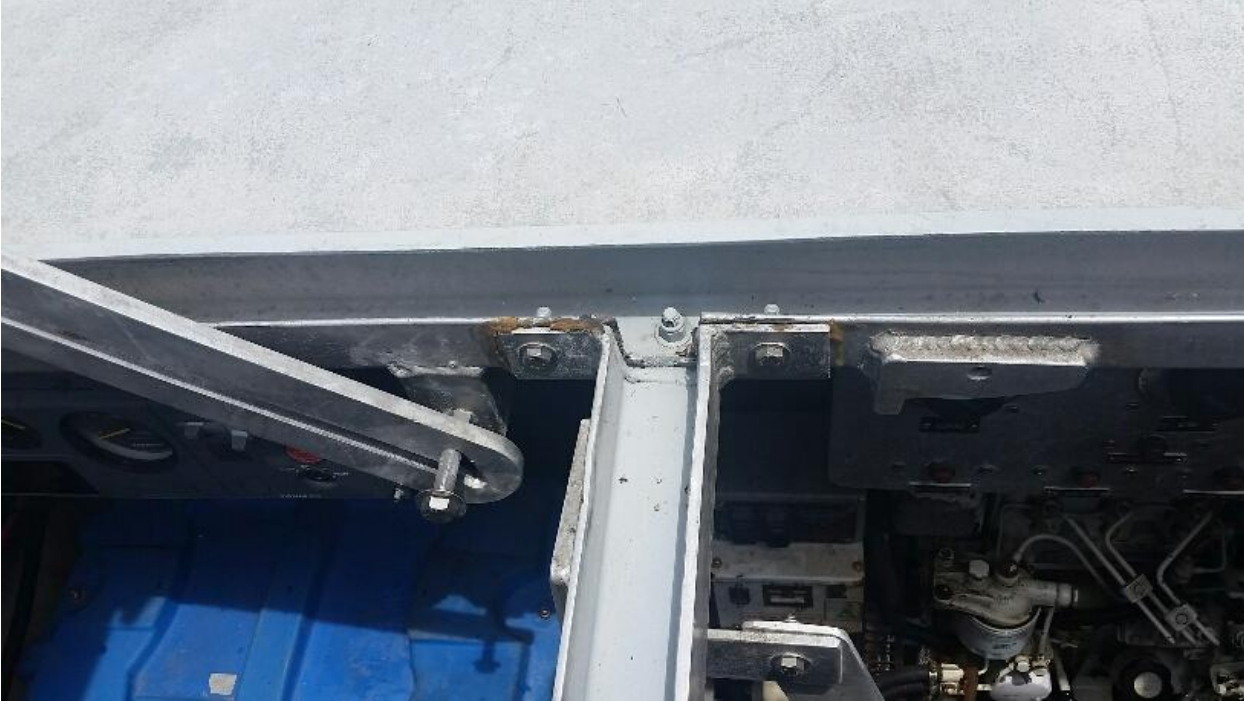
Hatch Brace Structure
